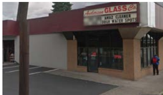
Wall 1 2516 E. Fourth Plain Blvd. - Anderson Glass Westside of building
