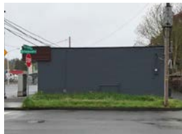
Wall 2 2818 E. Fourth Plain Blvd. - Grey Building Eastside of building
